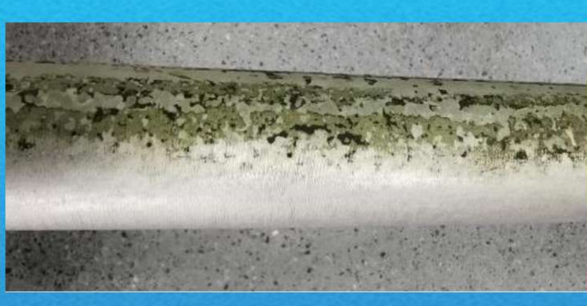
Cleaning of oxides and pollutants on the surface of steel pipes
